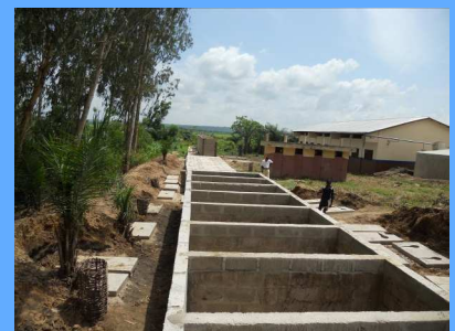
Construction of the toilets in Benin
