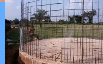
Rainwater tanks under construction in Nigeria
